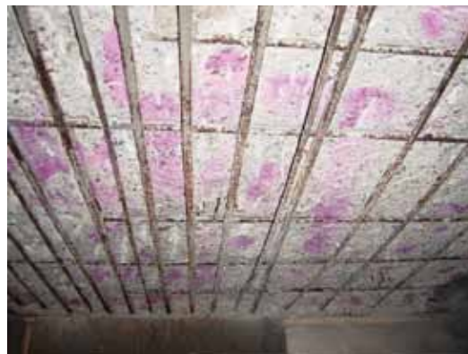
Fig. 6: Carbonated concrete removed and carbonation checked with phenolphthalein
