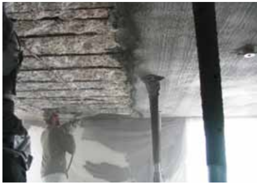
Fig. 7: Removal of existing concrete alongside completed shotcrete repair
