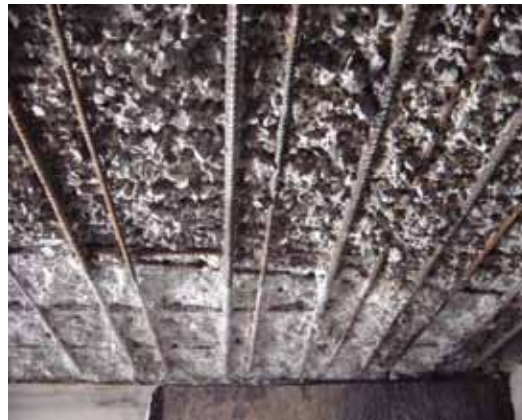
Fig. 5: Underside of roof slab illustrating difference between chipped area and hydrodemolition
