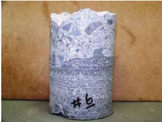
Fig. 8: Bond test core with failure within the substrate concrete
