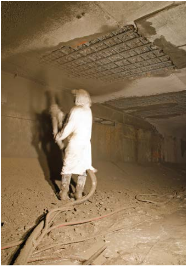
Fig. 5: Placing overhead wet-mix shotcrete
