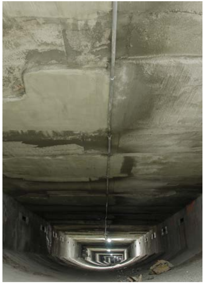
Fig. 6: Completed ceiling and wall rehabilitation
