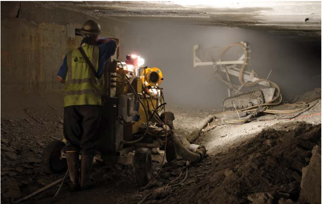
Fig. 3: Hydrodemolition robot in action removing overhead concrete
