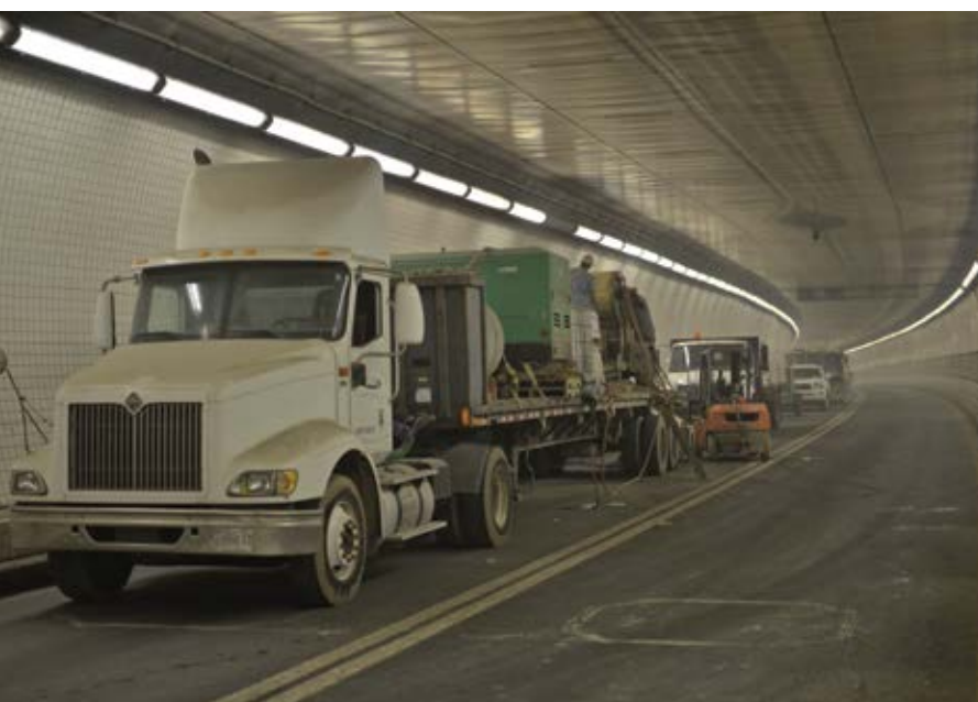
Fig. 1: Mobile shotcrete equipment in tunnel (work is underneath road deck)
