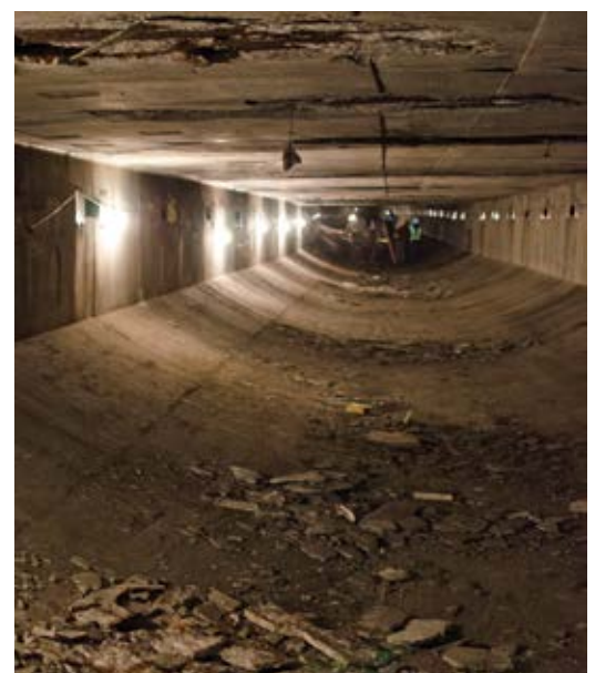
Fig. 2: Underside of road deck prior to rehabilitation activities
